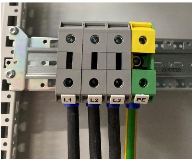
Figure 5-4: AC terminals on CombinerRack
