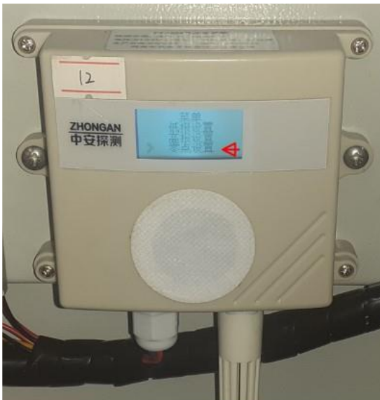
Figure 4-6: Zeroing the sensors
